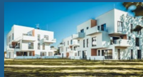
WROCLAW (PL) BACCIARELLEGO 54 (2ND CONSTRUCTION PHASE)
